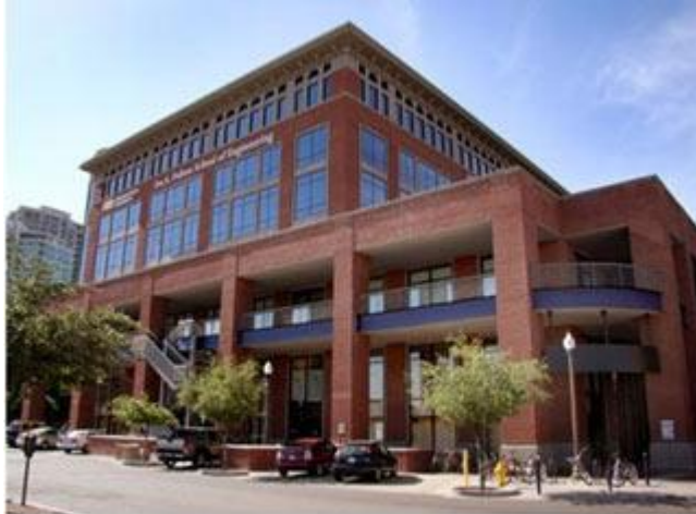
Arizona State University, Tempe Campus Brickyard Complex
